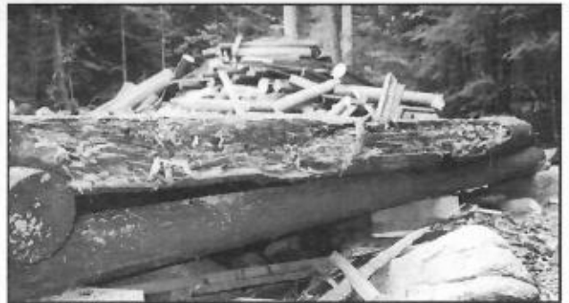
New #10 Cabin at Dacey Pond, shown under construction, above in a Bill Bentley photo, is larger than the old one and will hold six persons. At right, the Howard Lake photo shows a rotted base log, a prime reason for the replacement.
