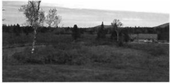
New construction at Nesowadnehunk Campground east of the stream Photo by Bill Bentley
