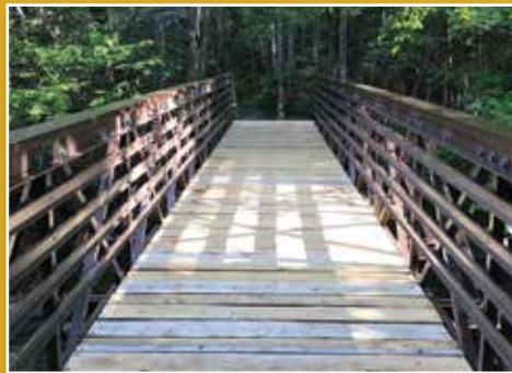
The newly-installed bridge over Roaring Brook features very durable materials and is expected to serve for 50 years or more.
