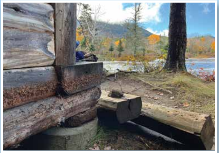
A waterline on lean-to #1 at Wassataquoik Stream on Saturday, October 15, 2022. Exceptionally heavy rainfall on October 14 caused widespread flooding in the Park and significant damage to roads and trails. – Photo © Aaron Megquier
