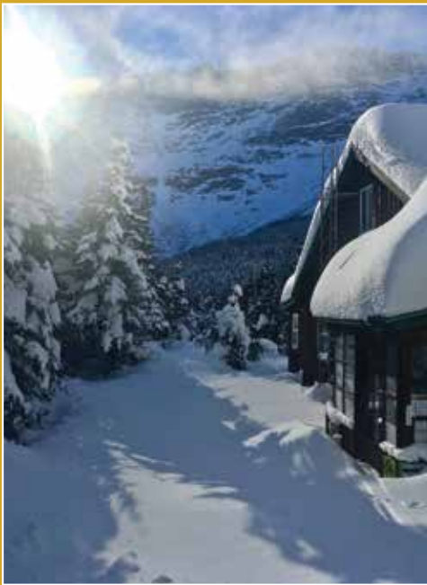
After sustaining flooding damage last spring, the Chimney Pond Ranger station was repaired over the summer and is back up and running. — Photo courtesy of Baxter State Park
