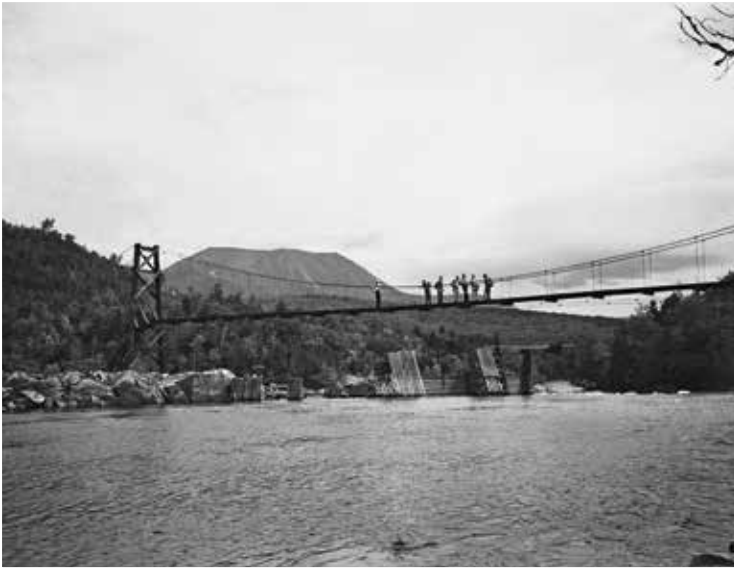
This suspension bridge over the West Branch of the Penobscot River was built in 1935-1936 by the CCC. It carried Appalachian Trail hikers over the river until 1963 – Photo courtesy Maine State Library, Myron H. Avery Collection
