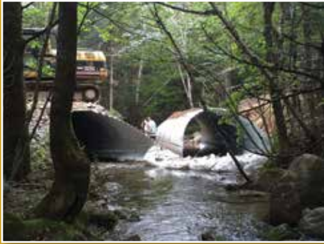
The culvert replacement project at Roaring Brook nearing completion.
