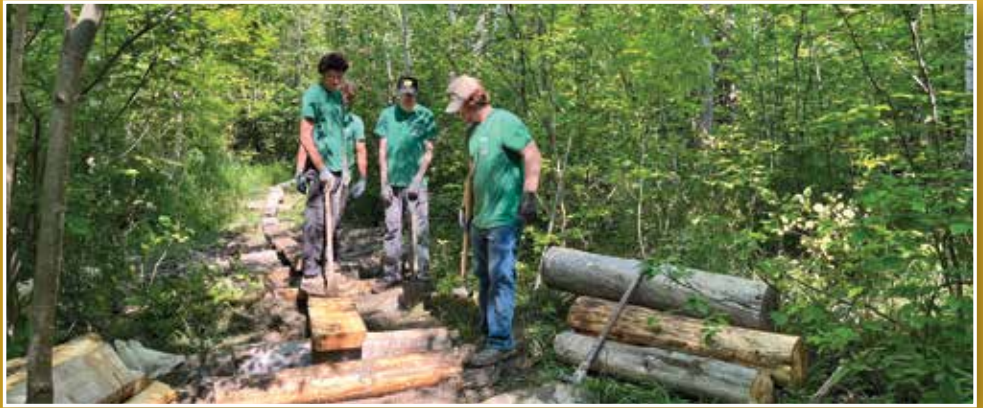
BYCC crew members working on a section of new bog bridging on the Pogy Notch Trail just outside of South Branch Pond campground.
