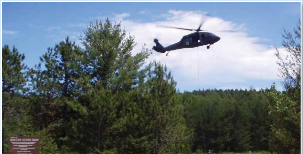
A Maine Army National Guard UH-60 Blackhawk helicopter picking up materials at Caribou Pit for transport to the new lean-tos being built on Wassataquoik Stream.
