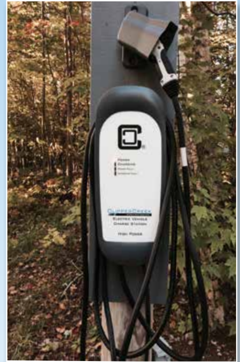
Baxter State Park's new electric vehicle charging station is located at Park Headquarters at 64 Balsam Drive in Millinocket, Maine. It is open to the public and features a J1772 plug.
