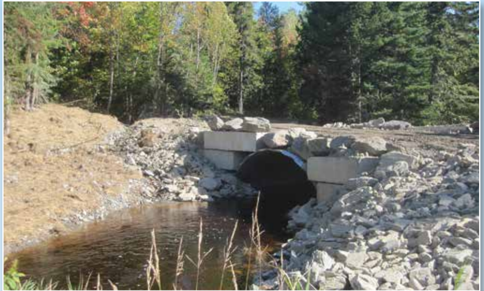
Black Brook Culvert
