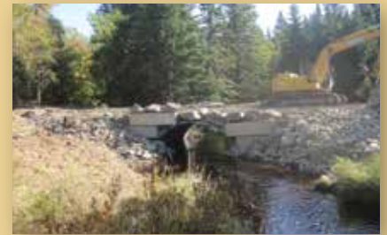
Black Brook culvert
