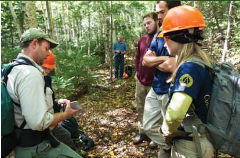
Maine Conservation Corps Field Team members take a break from trail construction on Mt. OJL to check in with BSP Trail Supervisor Paul Sannicandro. In background is Mick Rogers, Manager of Grants and Community Recreation, ME Division of Parks and Public Lands, on site to view progress on this project funded by Friends of Baxter State Park. – Photo © Bill Bentley
