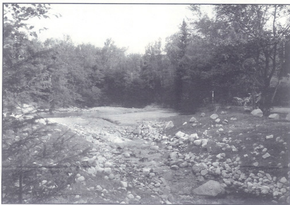
Dam Gone. This September '02 photo shows bank restoration at Katahdin Stream Campground following the removal of the dam. The smooth sand and gravel bars in the middle of the photo, deposited in the pond over the years, will probably disappear as soon as freshets scour the site.
